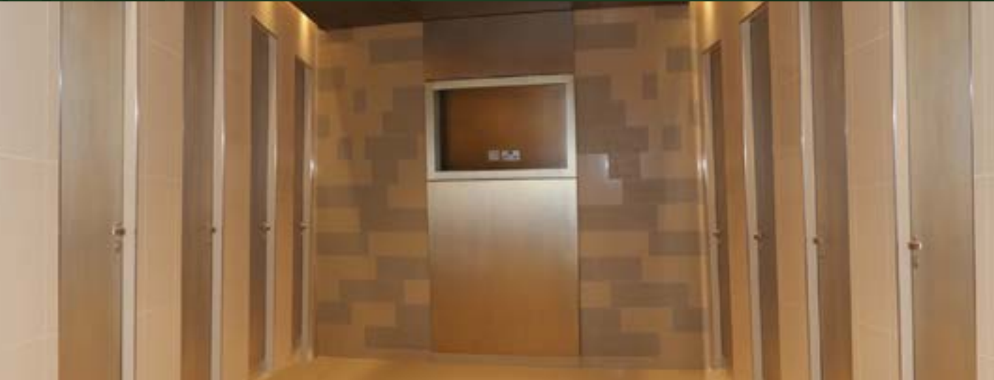
Electro Plating Cladding Works and SS Interior at Mall Of Emirates, Galleria Area
