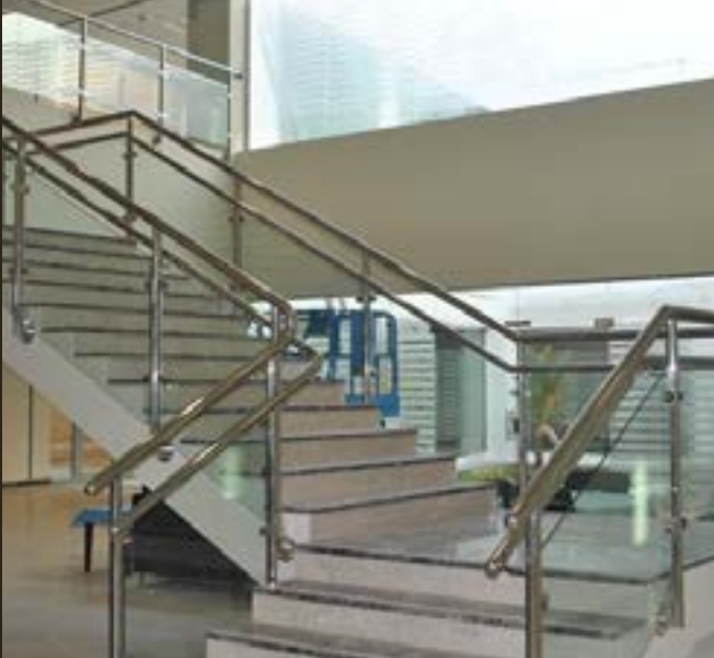
SS Handrail with Glass at Alain School
